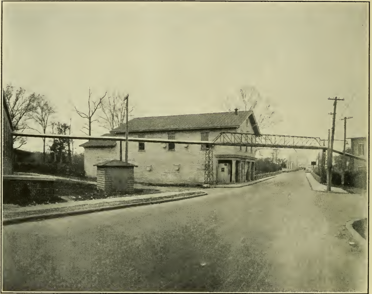
COTTON CONVEYOR PIPE TO MAIN MILL
