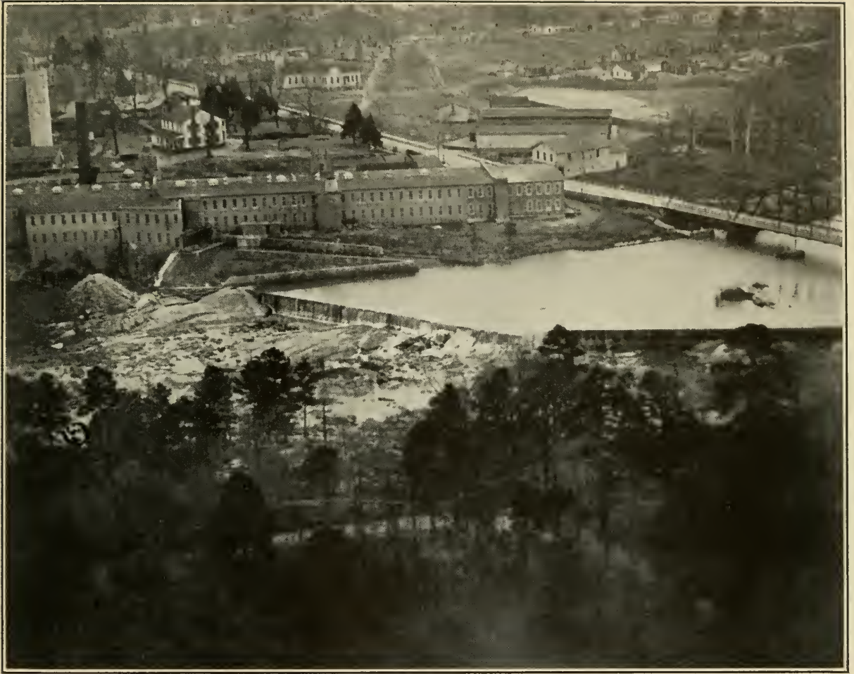
VIEW OF MILL, DAM AND SECTION OF VILLAGE
