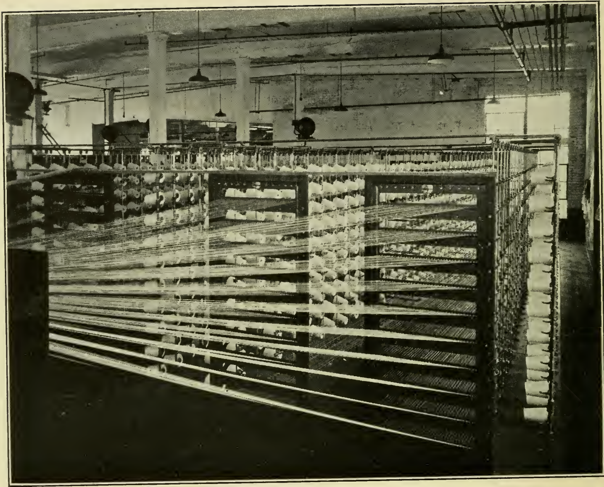
CONE CREEL FOR LARGE CAPACITY CHAIN WARPER
