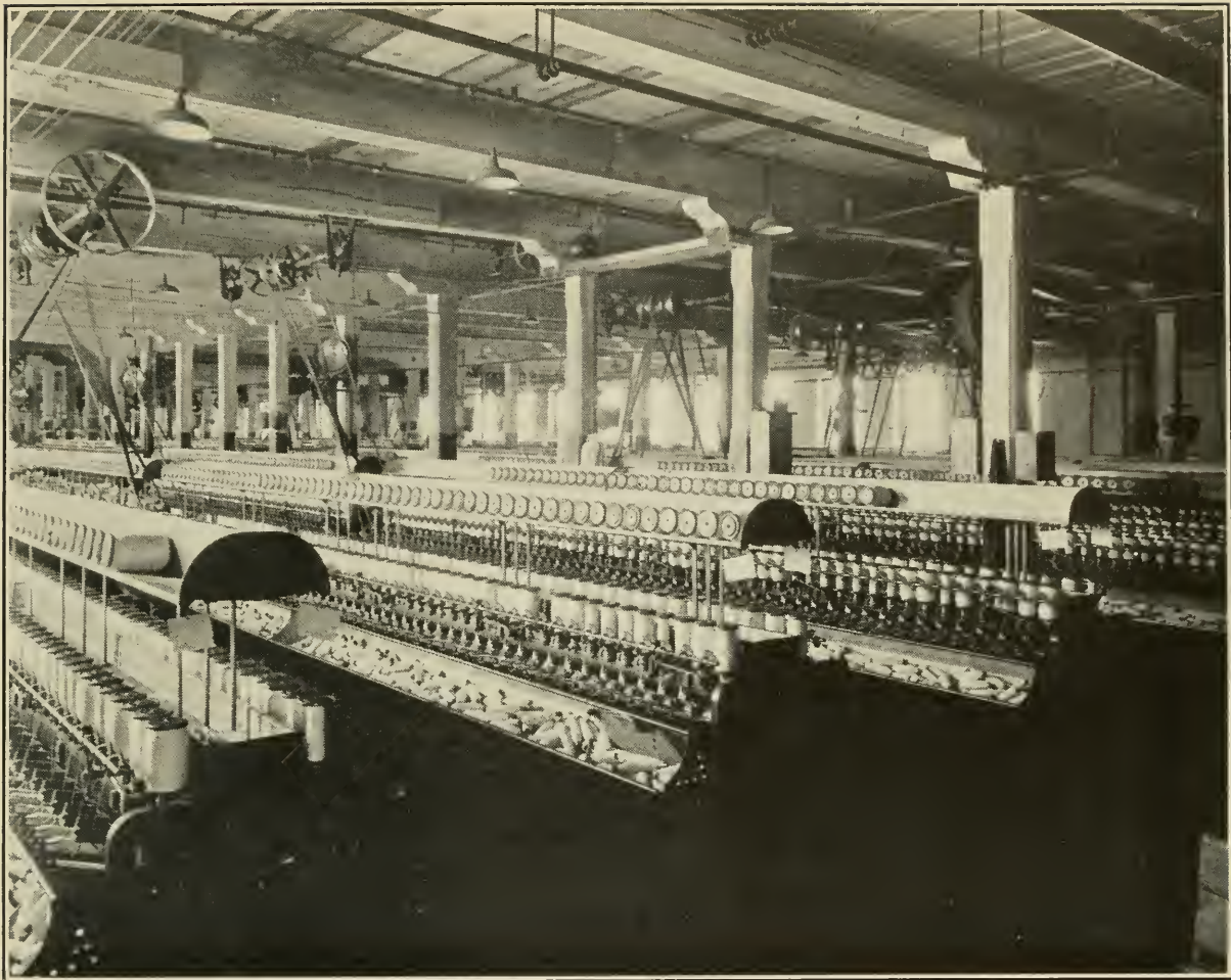
SECTION OF SPOOLING DEPARTMENT
